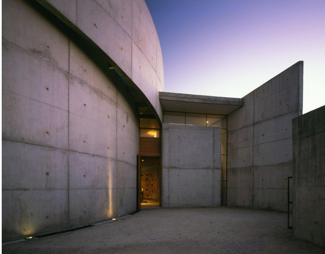
Second entrance, showing the weights, counter-weights and support of the building
