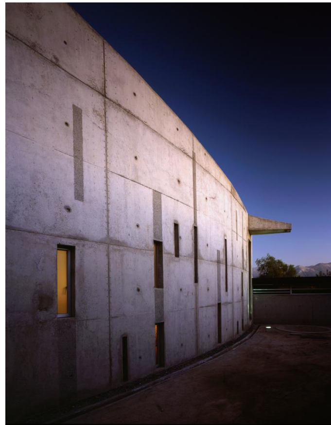
Side wall, confessional windows
